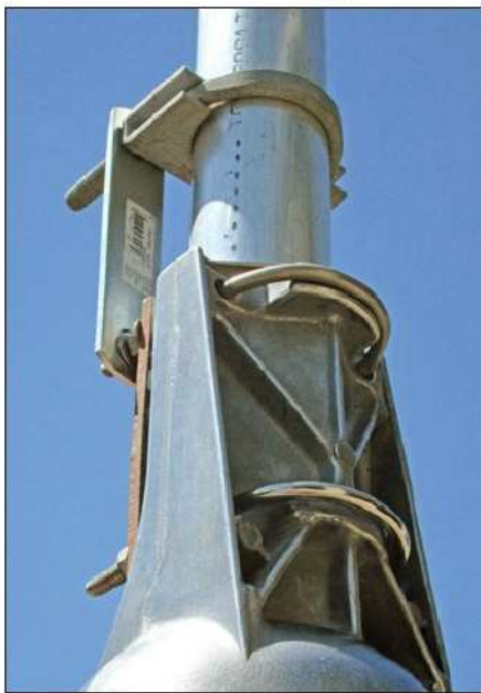
Figure 4 — A U-bolt with a flattened clamping area (A) for greater clamping force. [Photo courtesy of DX Engineering] A homebrew version is shown at (B) using a pair of straps to add a second clamp for extra clamping. [Don Daso, K4ZA, photo]
