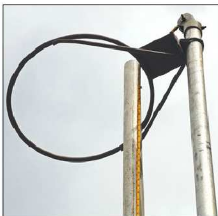
Figure 2 — A basketball hoop can be used with a gin pole to control movement as a mast goes into place. [Don Daso, K4ZA, photo]
