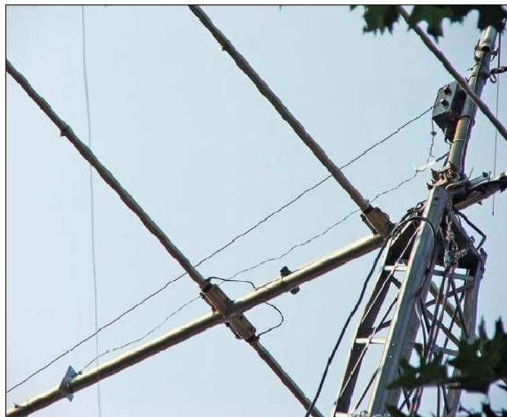
Figure 4 — Completed shunt assembly mounted above the boom and attached to the tower.
