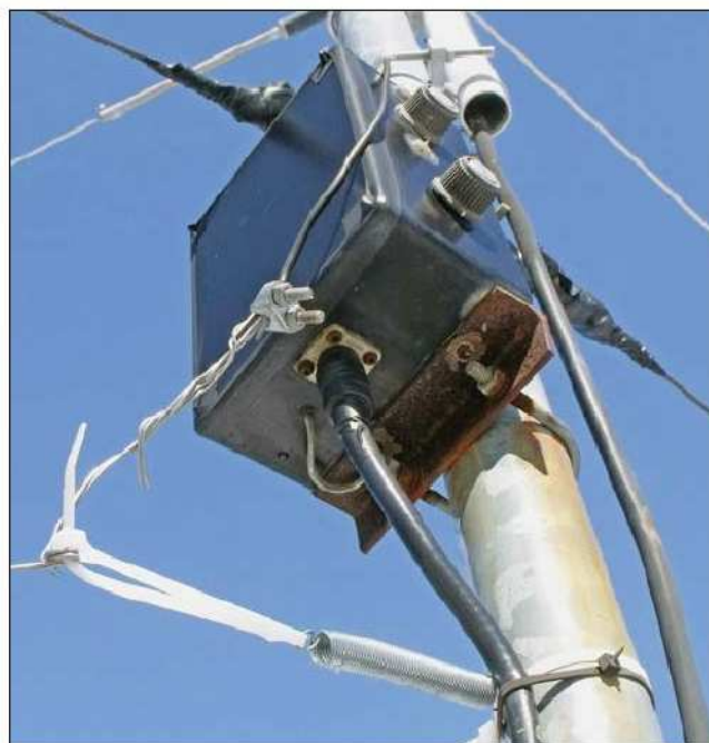
Figure 2 — The omega match housing attaches to the mast.
