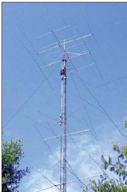
Figure 9 — RemoteHamRadio cofounder Ray Higgins, W2RE, works on the antennas at WebDX station in Monticello, New York. The antenna farm available to remote users includes monoband Yagis for 40 through 6 meters, a full size vertical for 80 meters and a 160 meter inverted V. [Photo courtesy Lee Imber, WW2DX]
