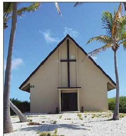
Figure 4 — This abandoned chapel near the ocean became the location for the two CW stations.
