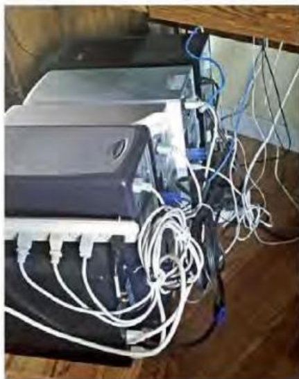
Figure 2 — A closeup of the pedestal swung out to the left, giving access to the backplane of all the equipment. [Dennis Merritt, W6UHQ, photo]
