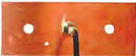
Figure 1 — The copper wall plate. [Lionel Booth, N5LB, photo]
