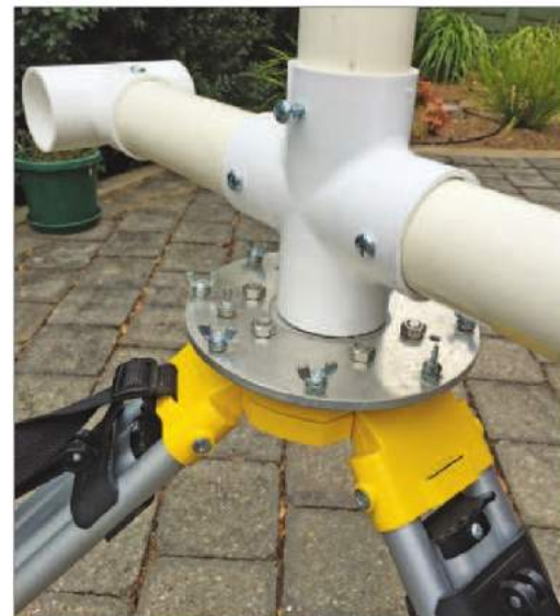
Figure 4 — A close-up look at how the joints are assembled. Riveting or screwing the joints avoids structural failure due to loss of glue integrity.
