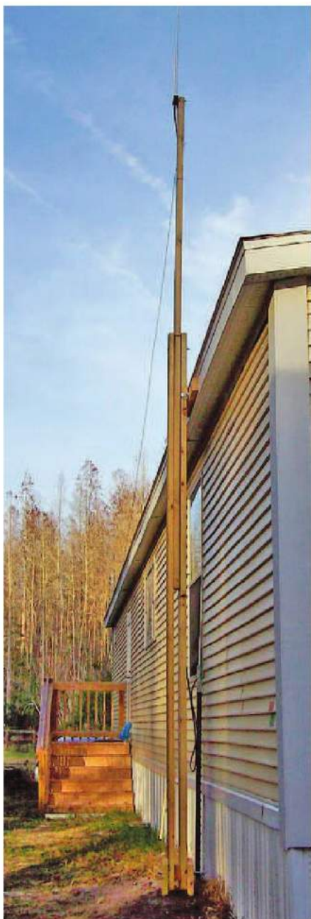
Figure 4 — The completed wooden antenna support. [Karl Schwab, KO8S, photo]
