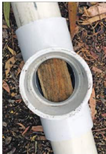
Figure 3 — Timber insert into the main vertical support. This hardwood pole adds stiffness to the structure.
