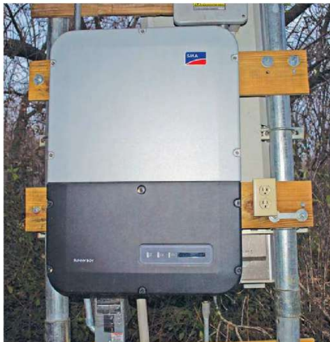
Figure 5 — SMA grid-tie inverters have an option for a grid-down secure power outlet that can provide up to 15 A at 120 V for power.
