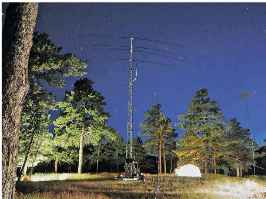
The Boulder Amateur Radio Club, WØDK, erected a 55-foot retractable tower in the Rocky Mountains in Colorado for 2019 Field Day. The tower supports a SteppIR three-element beam, along with a 30- and 40-meter loop. [Jack Ciaccia, WMØG, photo]
