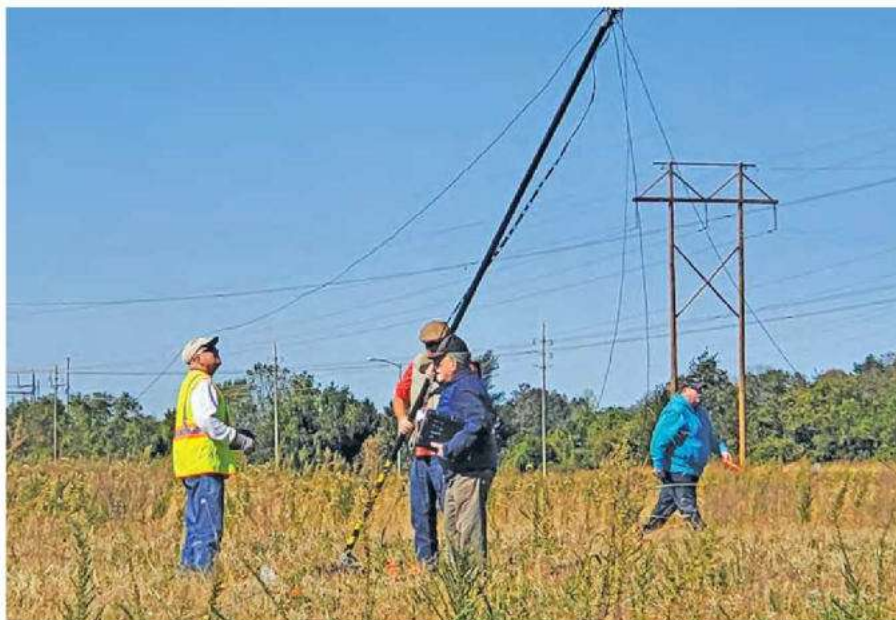
During the St. Charles County ARES SET, a team learned to assemble and test an NVIS antenna for a station within a communications trailer. Another team deployed a dual-band and a TV antenna for the station in the field under simulated emergency conditions. [William Grimsbo, NØPNP, photo]
