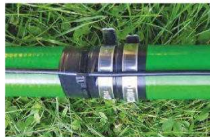
Figure 7 — Secure the junction of two sections of the antenna mast using electrical tape and hose clamps.
