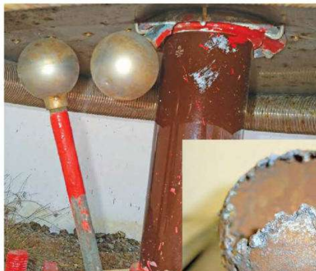
Two lightning corona discharge balls, used as lightning arrestors, placed at the base of the tower. [Andy Corbin, W4KDN, photo]
