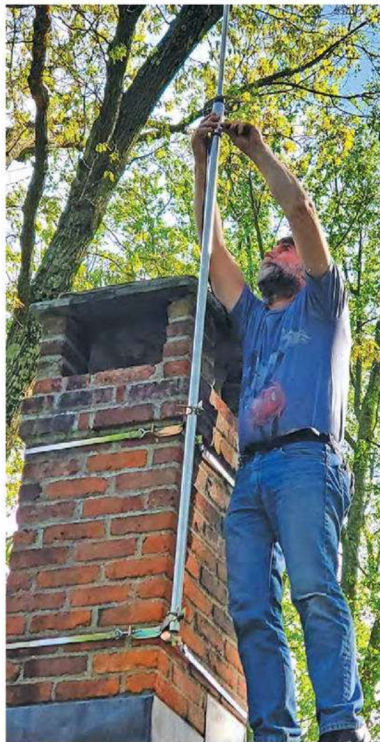
▶ Figure 12 — The author's son-in-law, Michael Phillis, finalizes the installation of the AR-2 on top of a 6-foot mast attached to a TV antenna-designed chimney mount. [Katie Phillis, photo]
