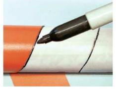
Figure 3 — Drawing the guideline for accurately applying the copper tape.
