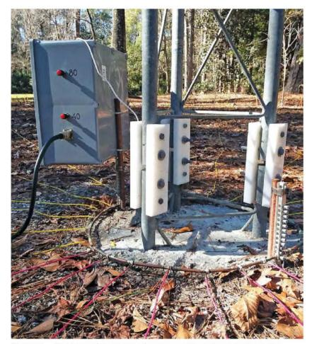
**Figure 4** — The base of the high-performance vertical shows the insulating base hinges, the matching network enclosure mounted on one of the ground rods, and a portion of the radial system.
