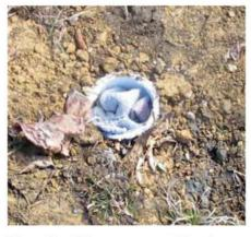
Figure 2 — Whenever you need to set up a temporary mast to adjust an antenna, simply remove the cap and slide the mast into the tube. [Robert Bastone, WC3O, photo]
