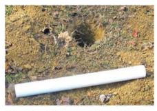
Figure 1 — Dig a hole at least 4 inches in diameter and bury a short length of 2-inch inside diameter PVC tubing. [Robert Bastone, WC3O, photo]
