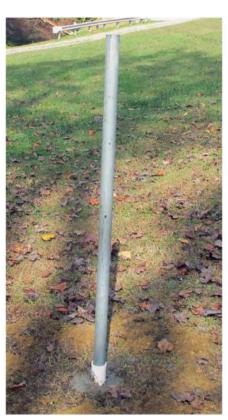
Figure 3 — Concrete should be poured into the hole so it surrounds the tube. [Robert Bastone, WC3O, photo]
