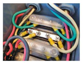
**Figure 5** — A close-up view of one of the bus bars with the cover removed. The copper bus bars are rated at 130 A and provide a safe connection point for the four conductors. [Paul Christensen, W9AC, photo]
