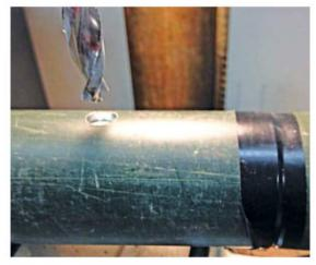
Figure 3 — Drill the hole through the female end of the mast by drilling through the existing hole in the male end.
