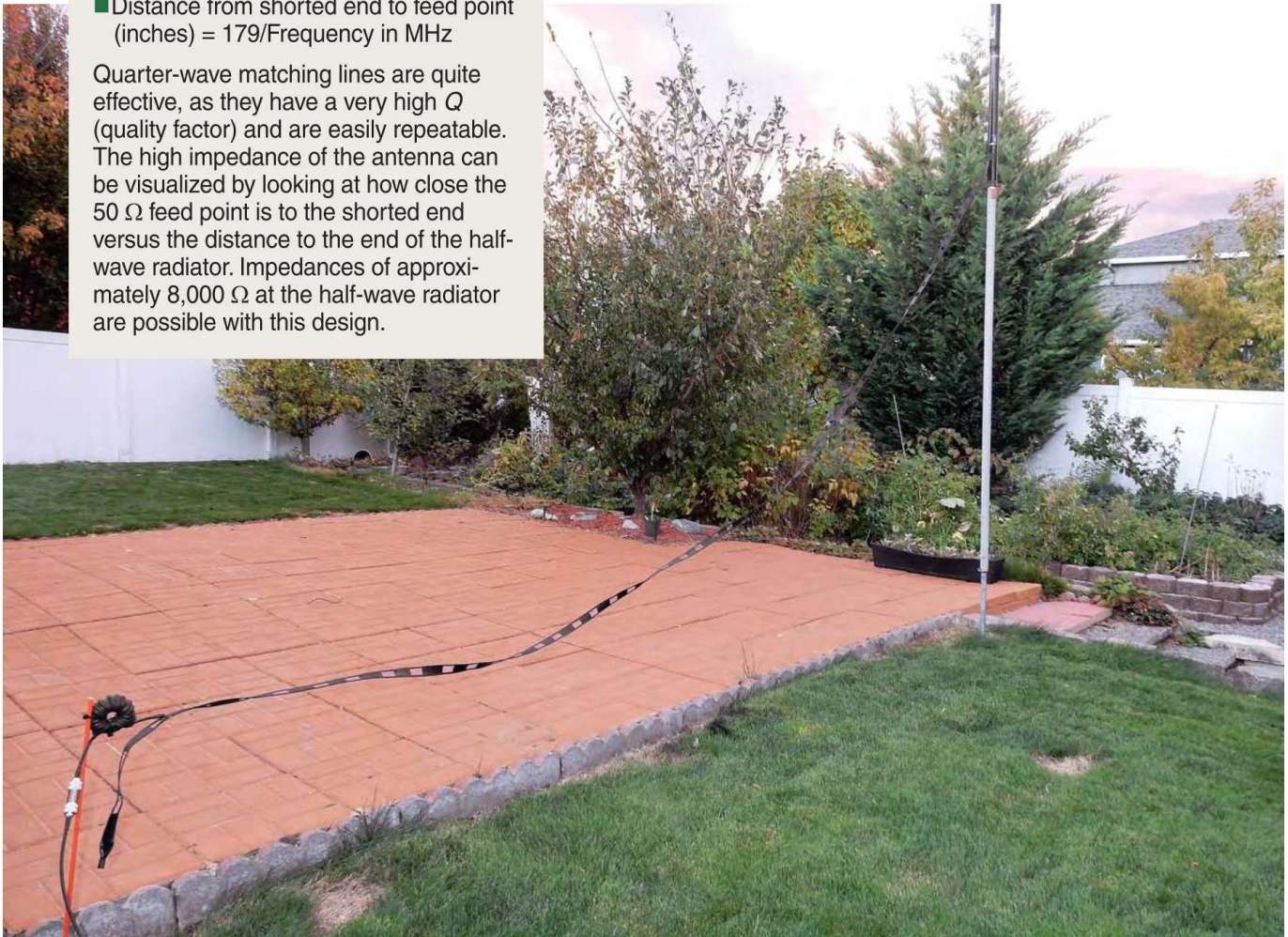
Figure 5 — The balun is supported above ground with a short pole.
