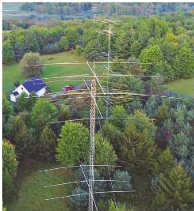
This RHR station in the Catskill Mountains in Summit, New York, offers 24 antennas across 24 towers for its remote operators. [Photo courtesy of Remote Ham Radio]
