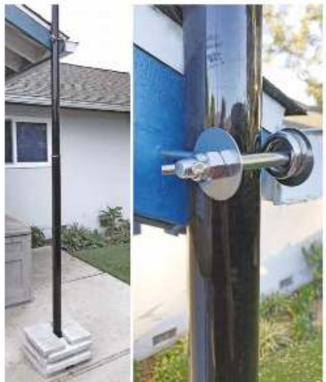
Figure 4 — What the mast looks like once it's mounted to the eaves. Note the stack of heavy patio bricks holding the mast in place.
