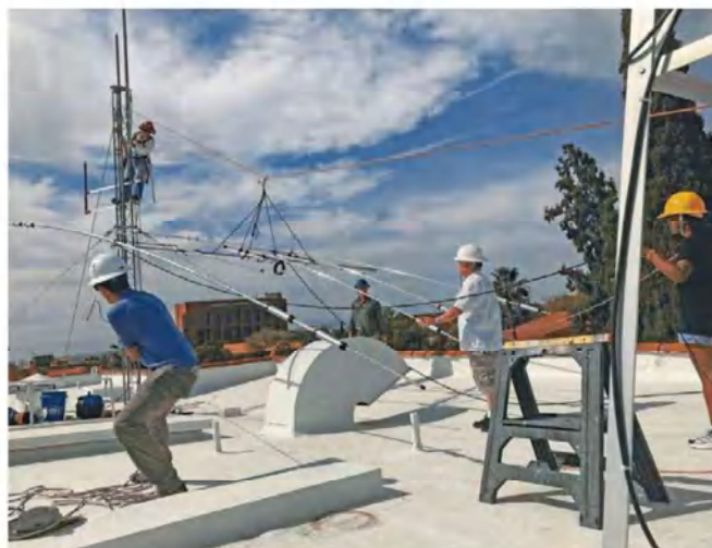
K7UAZ club members raising the new Mosley TA-63N antenna on the roof of the university's Old Engineering building, using an intricate system of pulleys and a tram line. [University of Arizona Amateur Radio Club, K7UAZ, photo]
