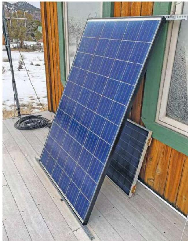
**Figure 2** — Dave's, KE0OG, solar panel. The charge controller reduces to the correct voltage to charge several AGM batteries that provide indefinite backup power to his radios.
