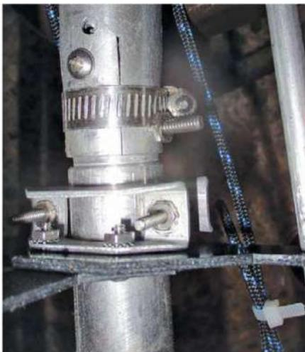
**Figure 1** — A close-up of one of the tube joints. Notice the stainless-steel bolts above and below the hose clamp.
