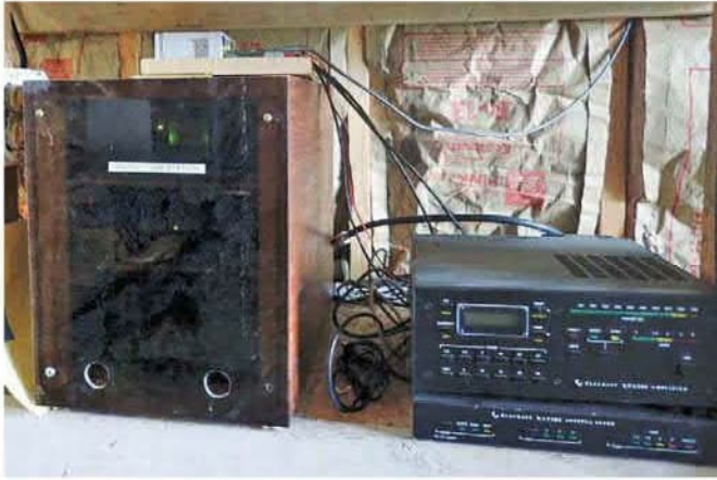
The Elecraft amplifier and antenna tuner are on the right. Dave Ingebright, WB7ELY, used the remote clients downloaded from the manufacturer's website to monitor the other equipment.
