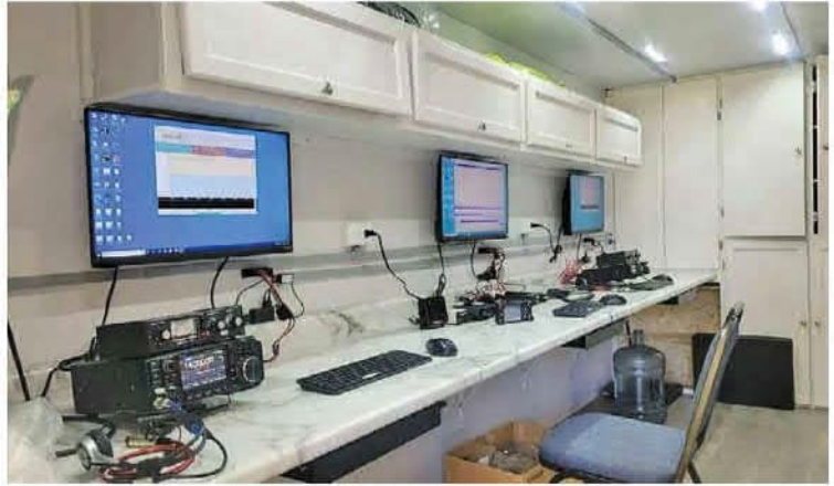
The inside of NIARA's fully equipped ham radio trailer.
