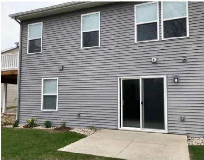
Figure 4 — The finished stealth antenna system. Look closely and you can see the antenna and ground lines exiting the patio door and the white self-adhesive clips carrying the antenna wire over to the connection at the downspout of the left side of the building. [Rich Barnett, N9NP, photo]
