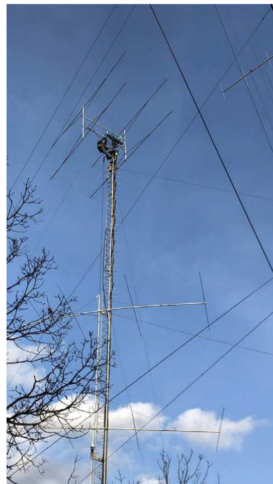
Dave Olean, K1WHS, performs pre-contest maintenance on his 222 MHz antenna array in preparation for the 2024 ARRL 222 MHz and Up Distance Contest. The antenna array consists of four 22-element antennas at 106 feet with azimuth and elevation rotation capability. [Dave Olean, K1WHS, photo]
