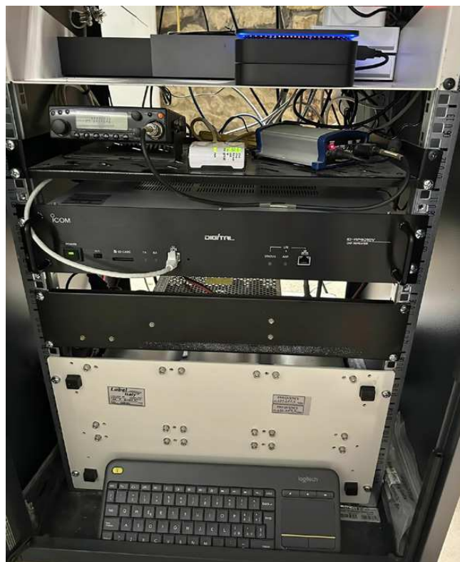
The new Icom ID-RP4010V repeater installation in San Marino. [Amateur Radio Association of the Republic of San Marino photo]
