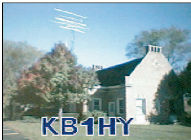
This view of W1AW was captured using a VC-H1. It was transmitted on VHF using FM and received on a second VC-H1 equipped station.
