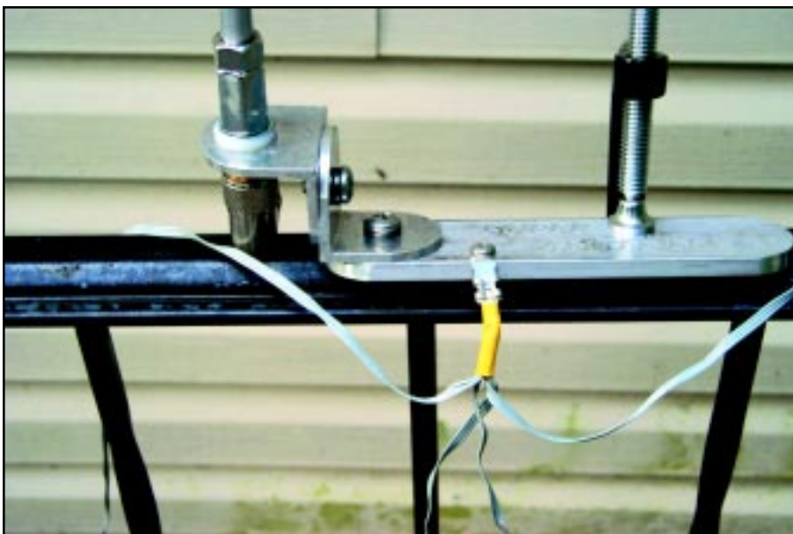
Figure 3 —A close up of the universal base. In this instance, the antenna system is attached to a balcony railing. The radial wires are spread out on the floor below.
