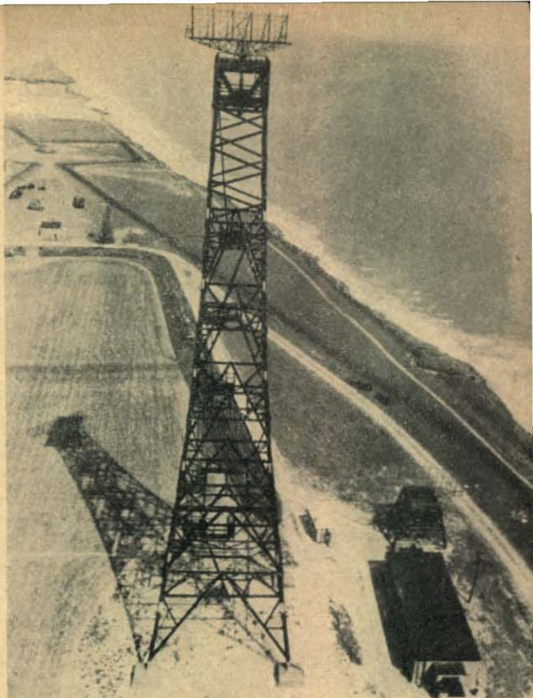
A "chain home low" radar station on the British coast. These installations detected low-flying planes. The five-bay four-stacked array is power turned atop a 185-foot tower. Should work nicely on the proposed 21-mc band!
