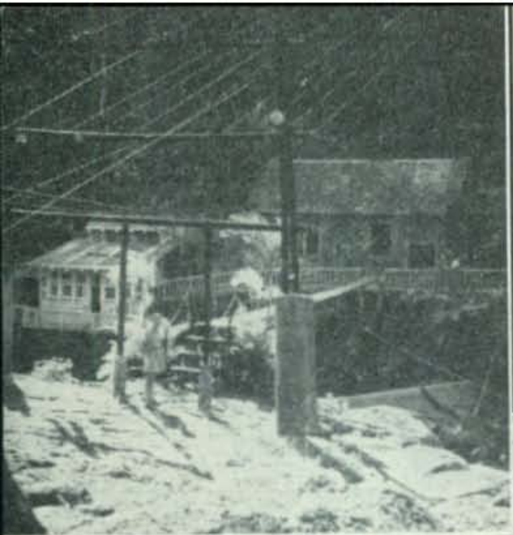
Redit hydroelectric power station built into one side of a ravine 300 ft. deep, showing VQ8AD standing before small suspension bridge.
