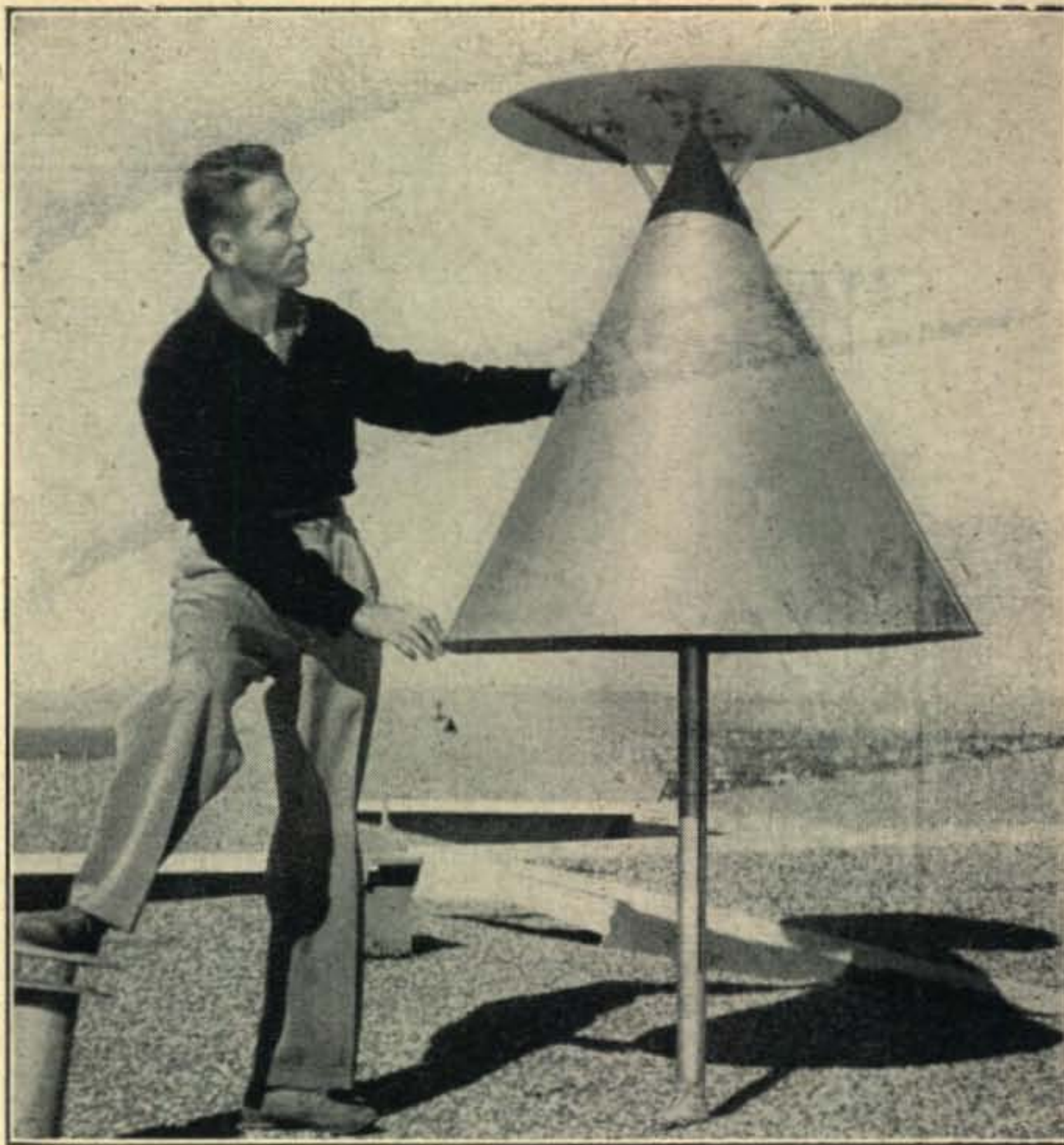
Fig. 1. W6UYH inspects a vertically polarized temporary test installation of the 40 to 500-mc discone.
