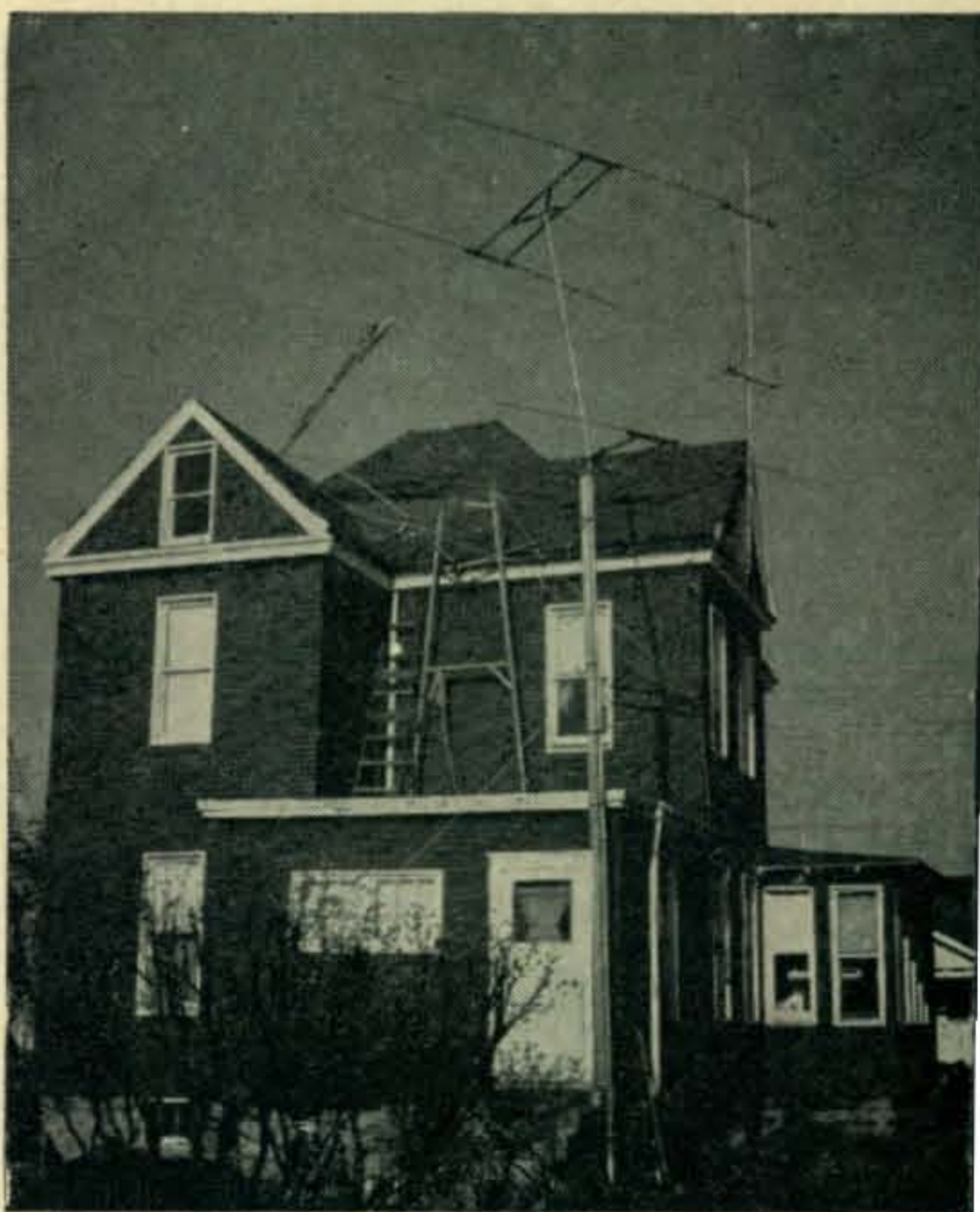
After the storm at W2PAU's. The ten and six meter antennas are left standing but the two-meter beam is gone over the edge of the roof!
