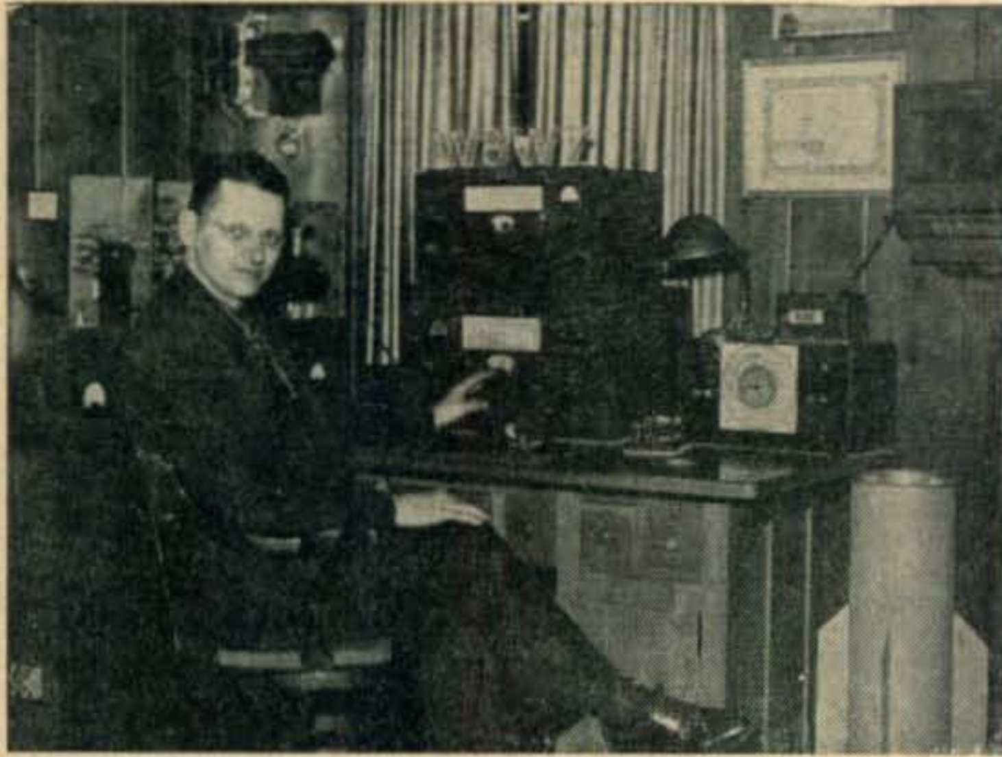
W8WZ scored 147,084 points. Doc runs a kw. into a pair of 250THs. Receiver is a 75A2. Antenna for 10-20 are 3 element beams, on 40 he uses 3 Bobtails, and on 80 a ground plane.
