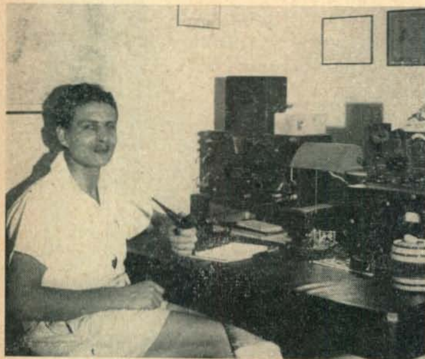
OQ5RA ran up 124,752 points. This was Andy's first contest since becoming a ham May 2, 1948. Rig uses a pair of 807s, 75 watts. Receiver is a BC-342.
