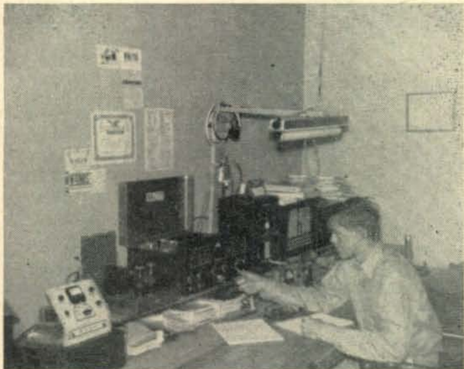
David Langley, of Aurorar, N. C., at the controls of WN4YDY. The transmitter is a Harvey-Wells Deluxe, with fifty watts input on the 3.7-Mc. band. The receiver is an SX-71. Dave made his first contact last Christmas day.
