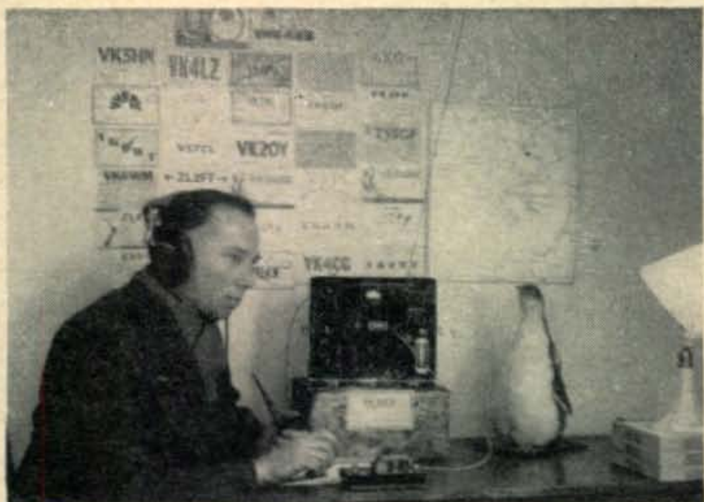
This photo was taken on December 18, 1948 when Allan Campbell-Drury, VK3ACD celebrated his thirtieth birthday. The occasion merited the donning of a full-fledged civilian suit (the first time in his 12 months at bleak Heard Island). The transmitter-receiver unit is a war surplus Type III Mark II with a power of about 4 watts into a length of wire.
