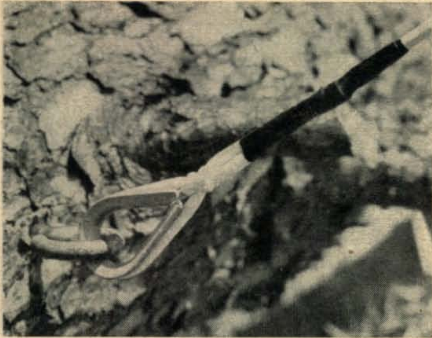
View of an open thimble and eye bolt for coupling the Glas-Line guy wire to a tree.
