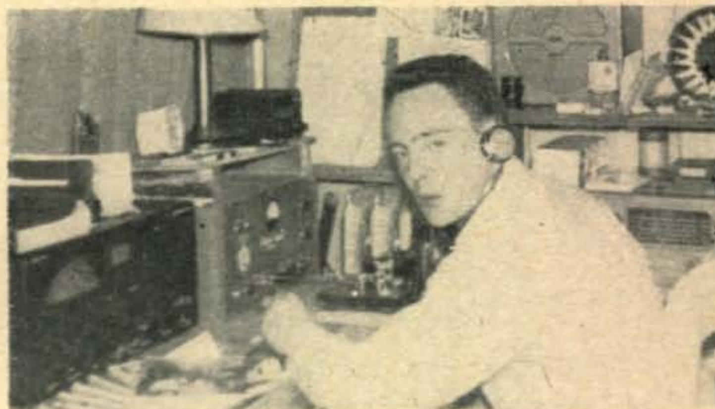
Sixty-five watts to a Globe Scout transmitter, abetted by an NC-98 receiver and a 75-foot antenna has earned Dave Corsair, KN2KHZ, Newark, New Jersey, 21 states and Canada in a few months on 80.
