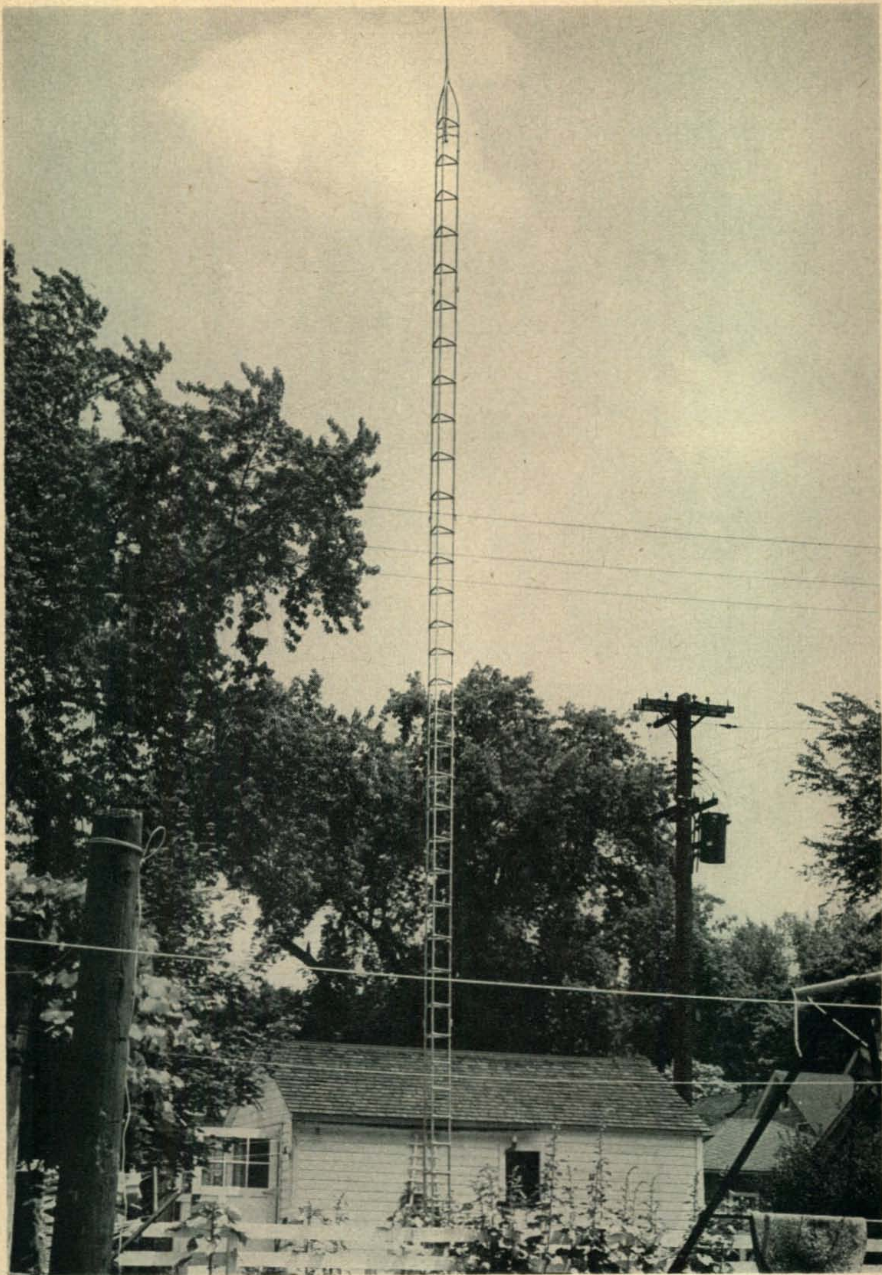
TV-tower antenna at W9UA. Aluminum tubing extends 32' above top of tower for a total radiator height of 82'. Entire structure is self-supporting.
