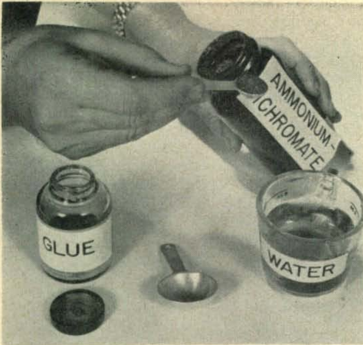
Fig. 4. Preparing the sensitizer.
