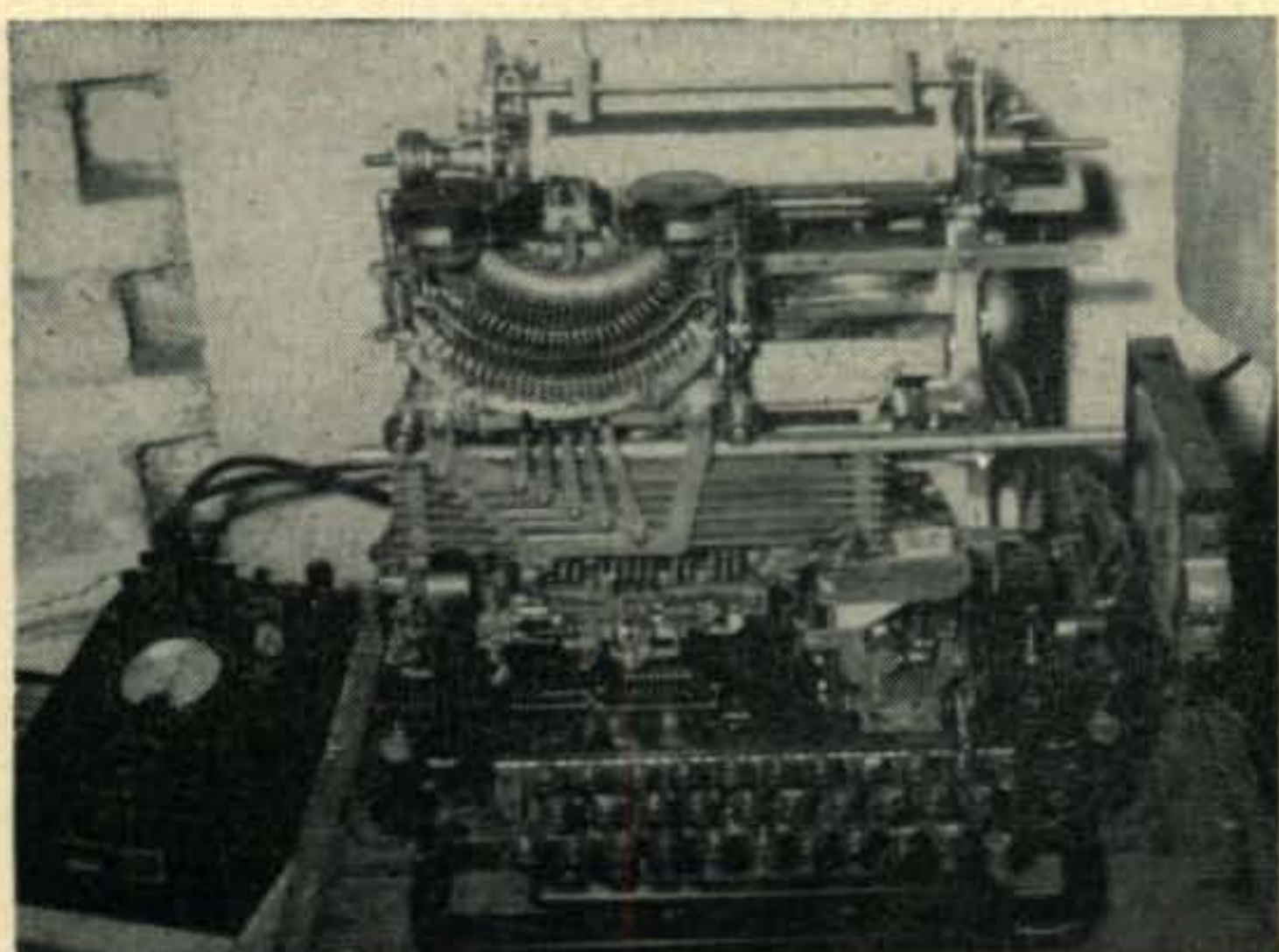
Model 15, Cover Removed; Line Unit BD-77-A to the left.
