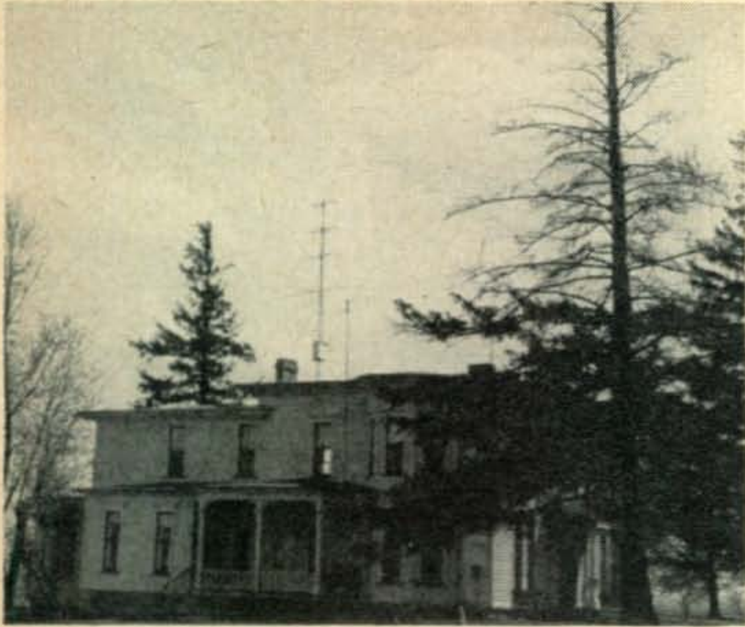
2 and 6 meter installation at W2UTH. 2 Meter beam is W3GV array.
