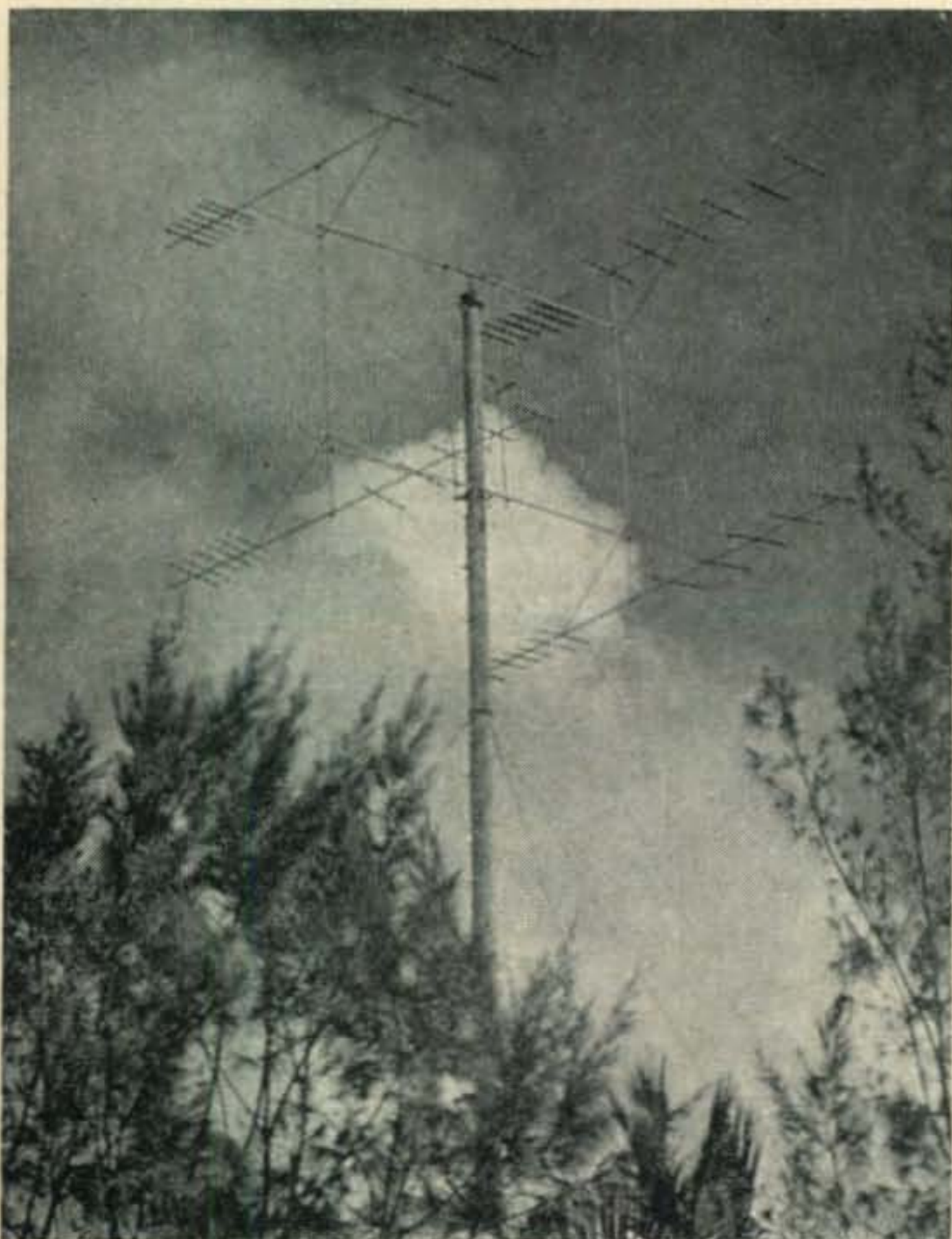
52 element 2 meter beam in place on top of 80 foot pole at KH6UK.
