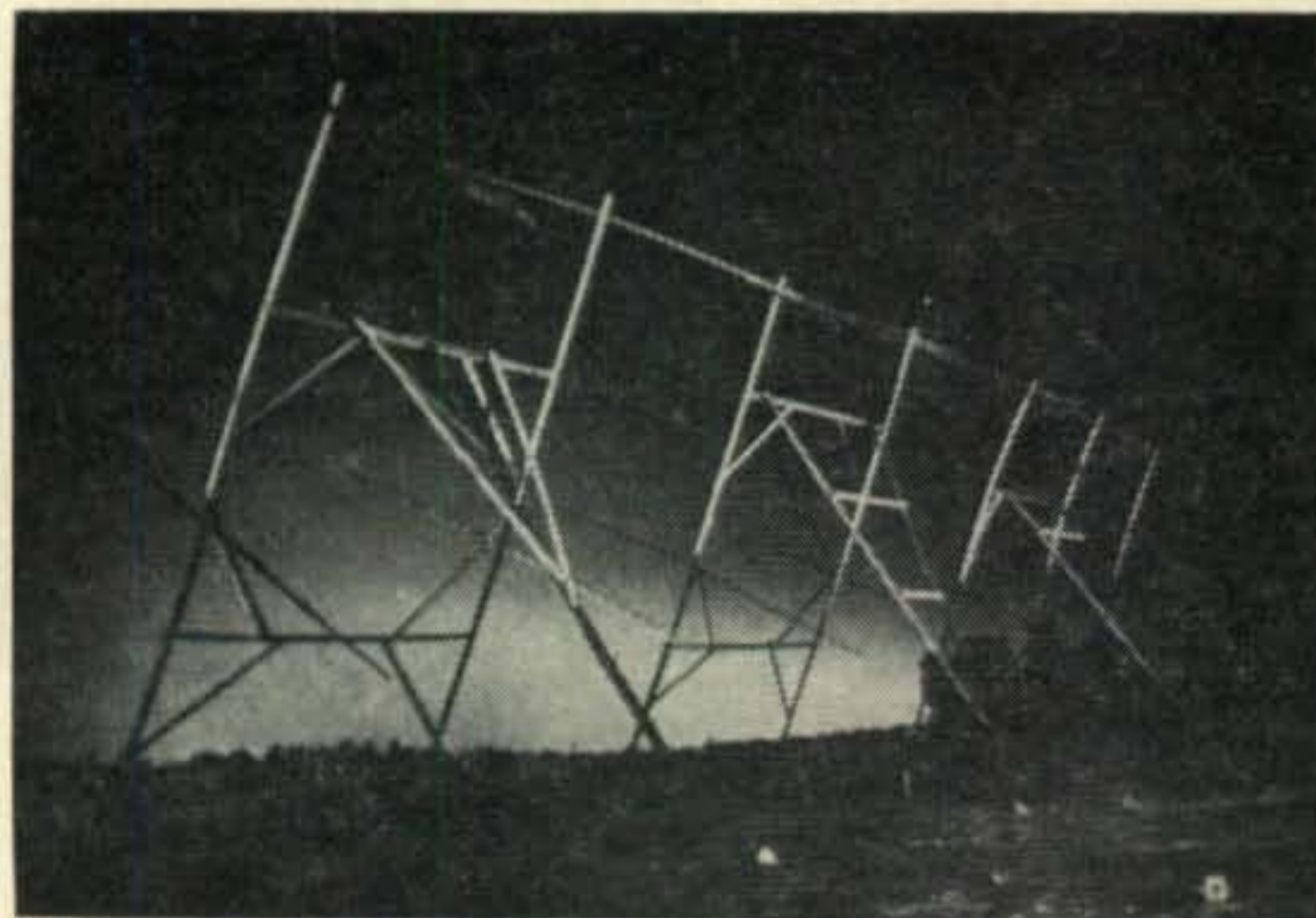
San Fernando moon beam. 16 Yagi's 13 elements each on 24 foot booms. 112 feet wide.
