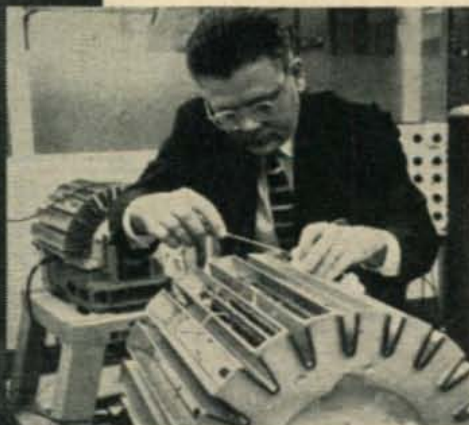
Dick trouble shooting Magnetic Drum Frame.
