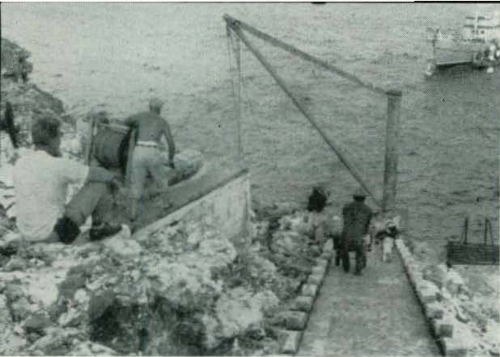
The heavy stuff was pulled up by winch and davit. Don watches George cranking up a load.
