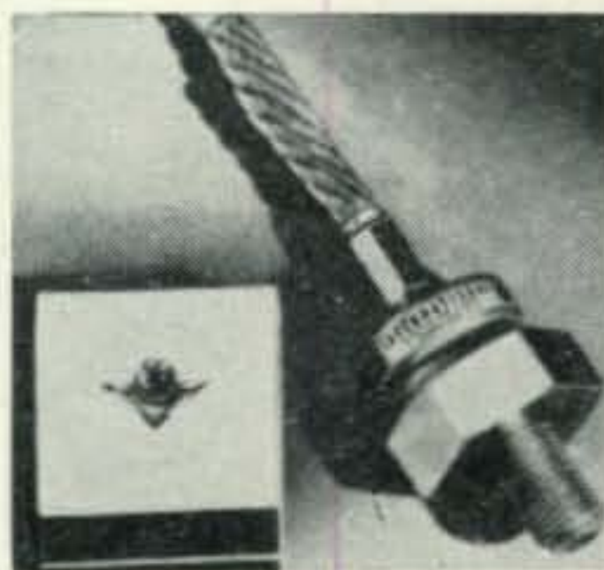
This silicon solar module, manufactured by International Rectifier Corp., can convert sunlight directly into electricity with conversion efficiencies in the order of 8%.
