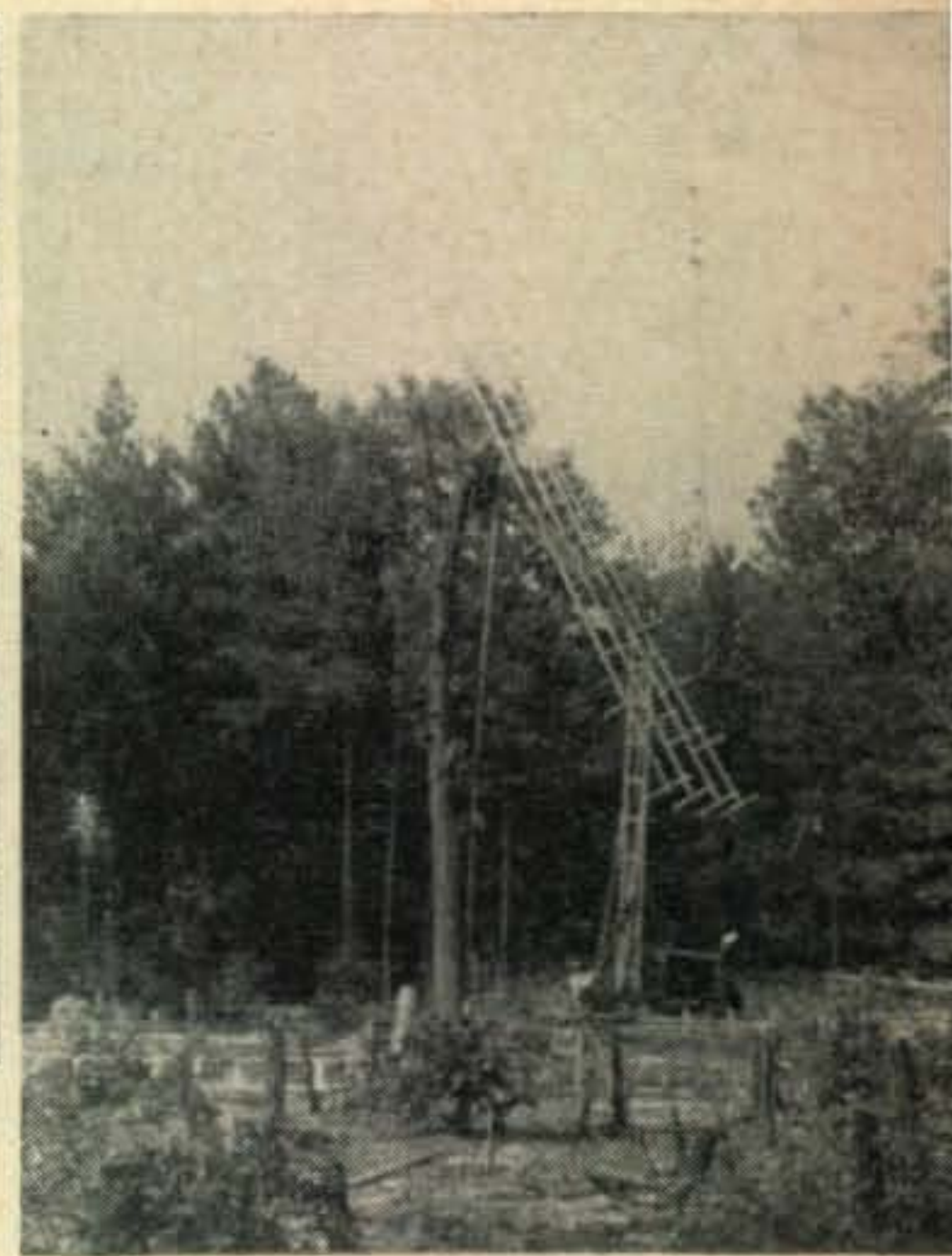
End view of complete system.
