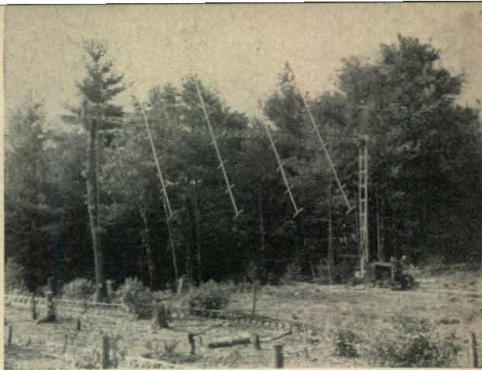
Overall view of complete installation.
