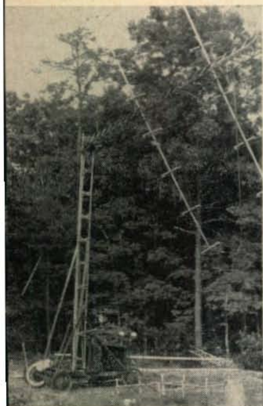
Side view of truck tower supporting outward end.
