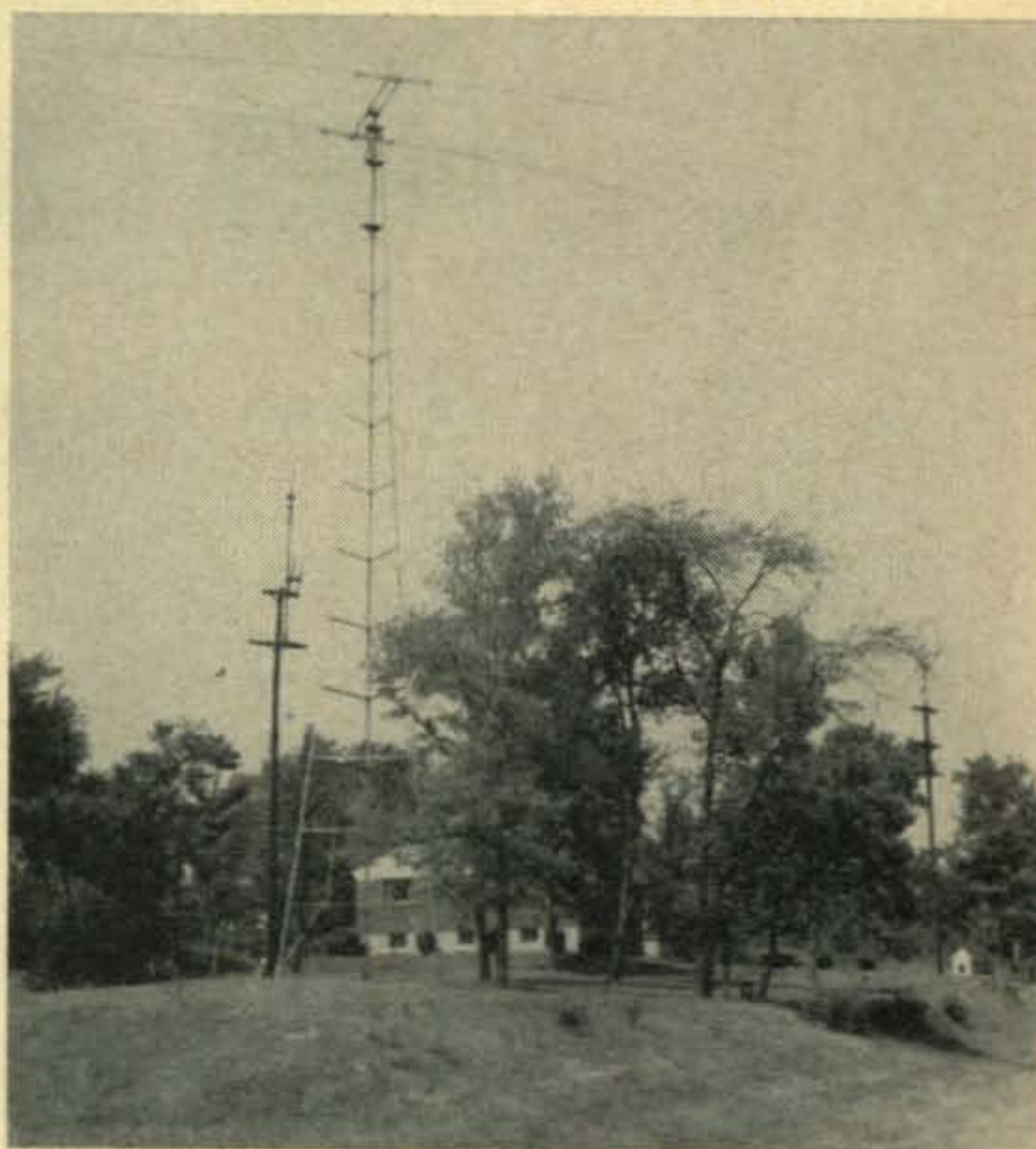
W8FGX's 7 mc rotary, full sized and 87 feet high. Does this explain Jake's potent signal on 40?
