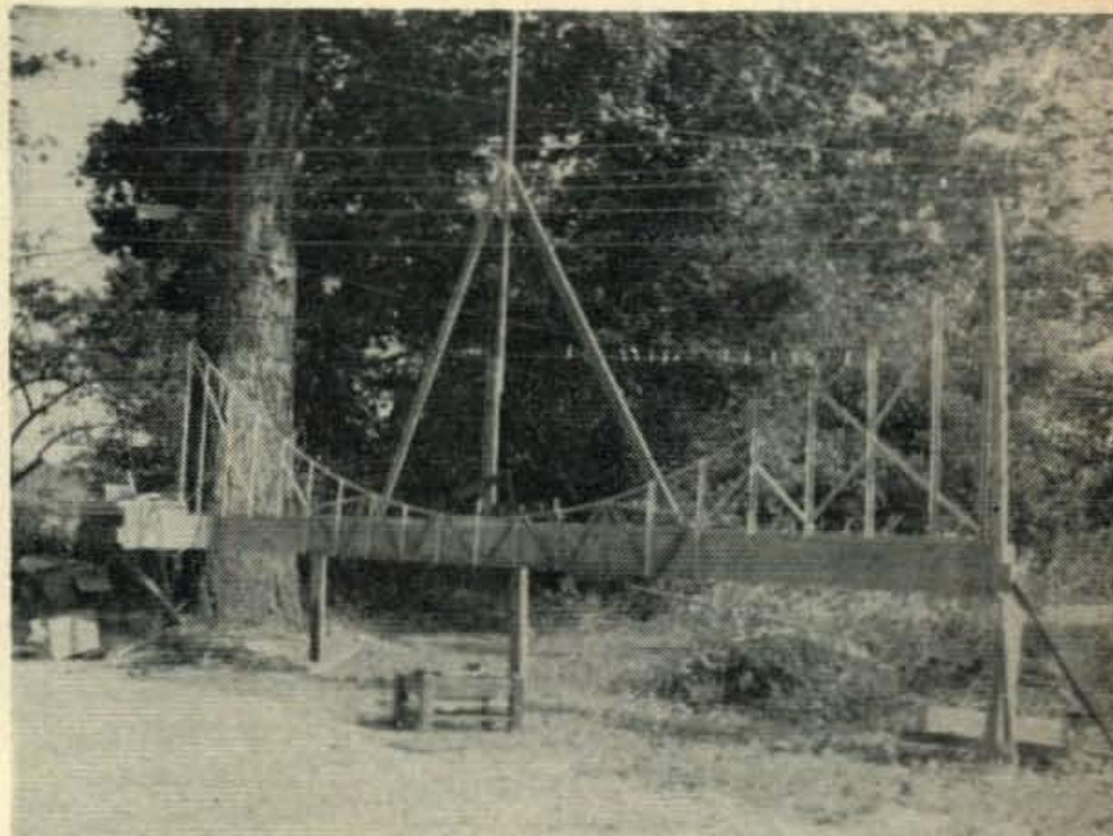
First completed section of parabola
