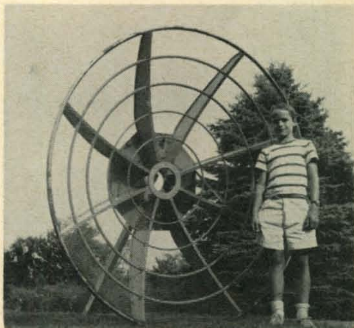
K1AUD's new 6' dish for 3,500 mc. Wayne wants me to mention that the boy in the picture is NOT K1AUD—hi!
