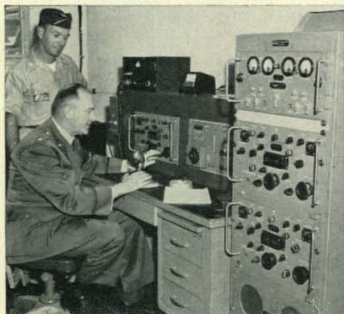
Col. Brundyge and Capt. Groves officiate at the opening of BV1USG. The station will be operated 16 hours a day and a training program is under way for new operators.
