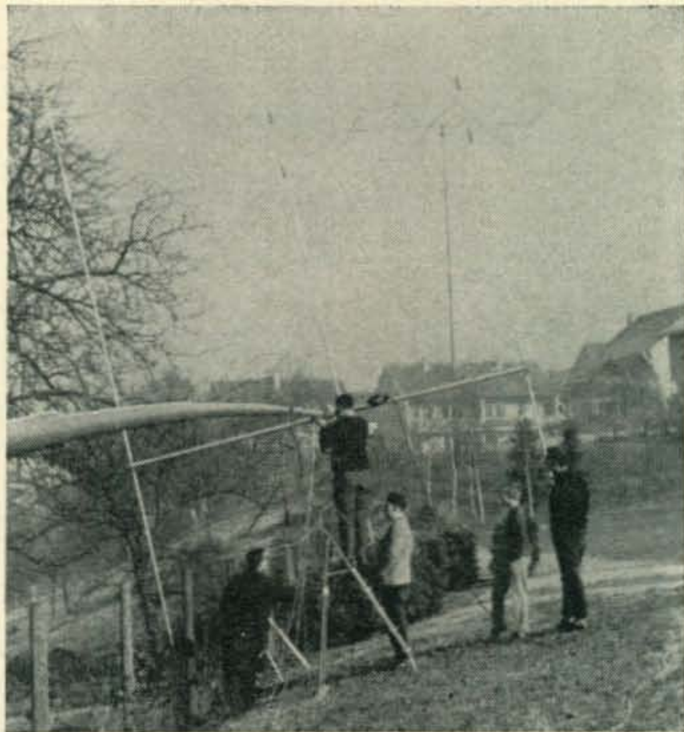
The DJ3JZ Gang preparing for the c.w. week-end. That's a tri-bander going up, adding to the extensive antenna farm needed for multi-transmitter operation.
