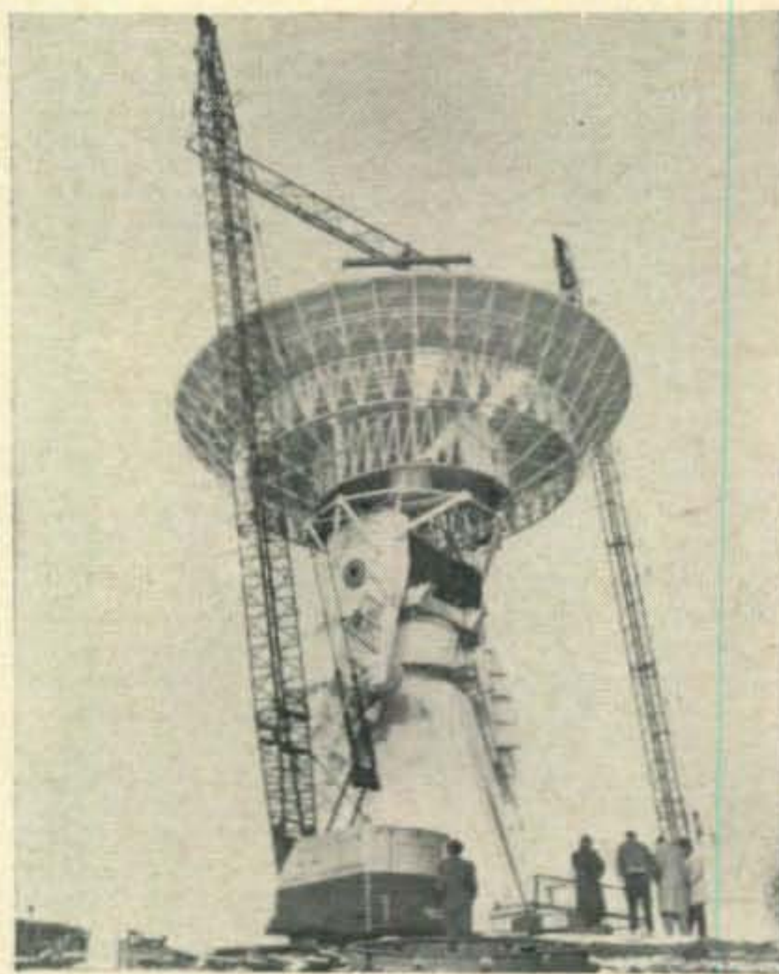
ADVENT parabolic dish antenna being installed at Camp Roberts, California, for communication with the "stationary" satellites.
