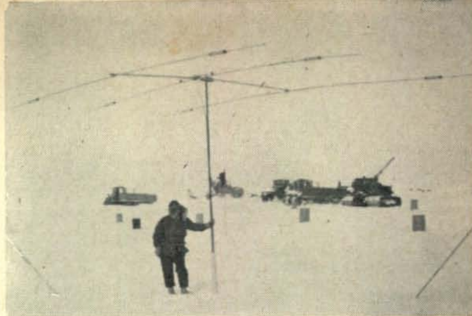
Forty feet below the surface lies KG1CC. Here, the author poses with the TA-33 which withstood winds in excess of 85 knots.
