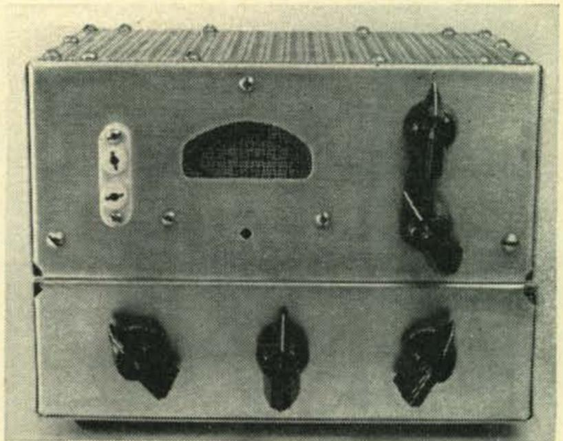
Front view of the six meter transmitter shows enclosure construction and placement of the various controls. The base of the unit is a standard 5 × 7 × 2 inch aluminum chassis, and the upper compartment is a 5 × 7 × 3 inch chassis. Controls from lower left to upper right are the Crystal-V.F.O. switch, Meter switch, Mode switch, Pi-network Output capacitor, and Plate Tuning capacitor. The meter is sub-mounted behind a piece of aluminum screen.
