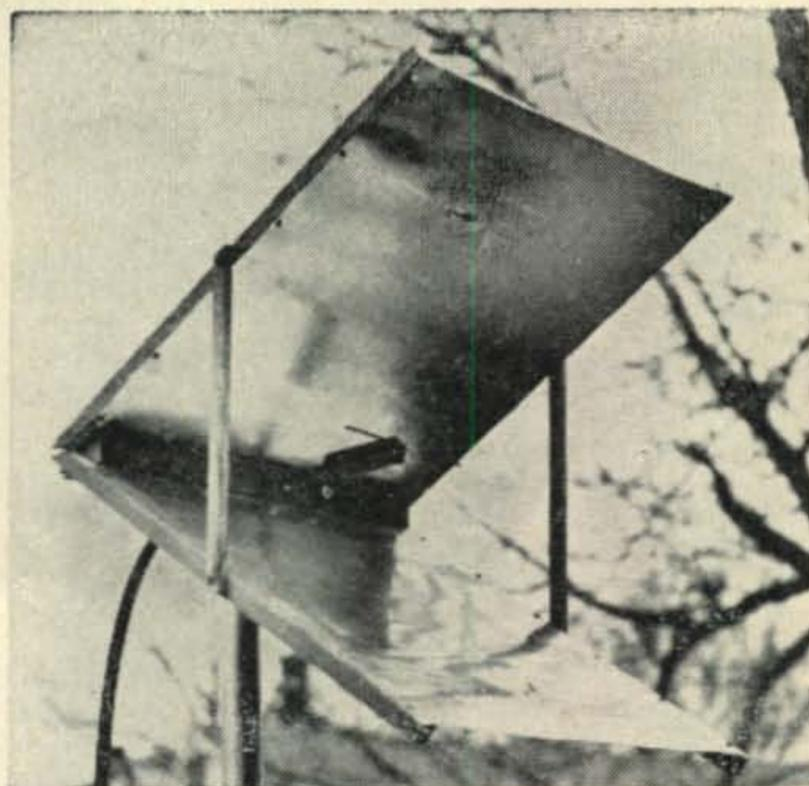
Simple 1220 mc corner reflector antenna at K2RGF.
