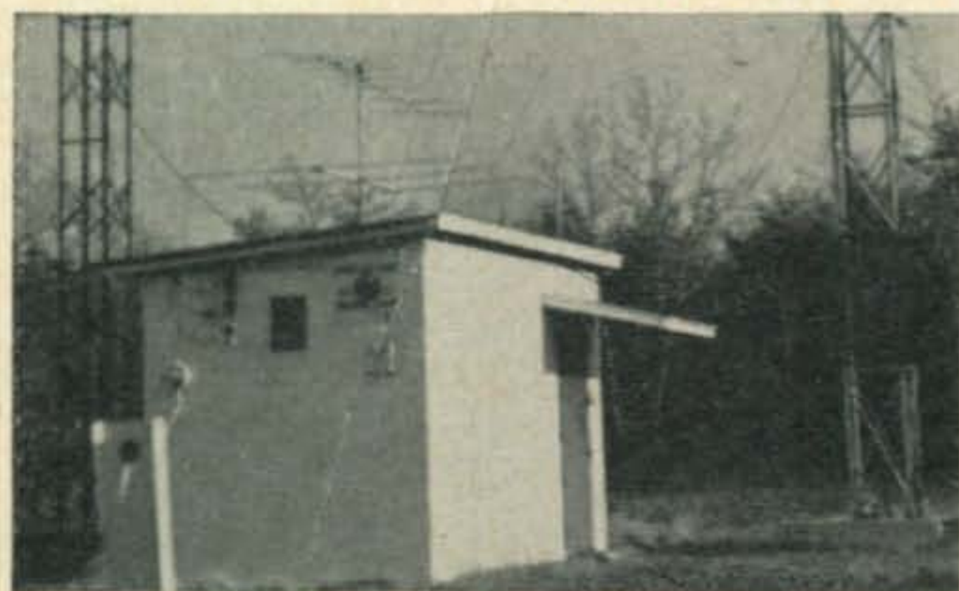
Commercial Broadcast station? . . . No. Those two towers (75' and 100') support the VHF antennas at W3HCW, Williamsport, Pa.
