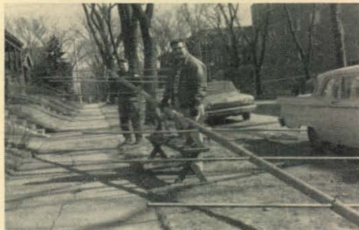
WA9FPC and WA9IMR repairing the 30 foot monster at W9JFP, Milwaukee. This six meter baby now weighs 90 lbs. (with "repairs") but it is still performing from atop Vic's 105 foot tower like always. Look for W9JFP/7 in Nevada on the 13th and 14th of June.
