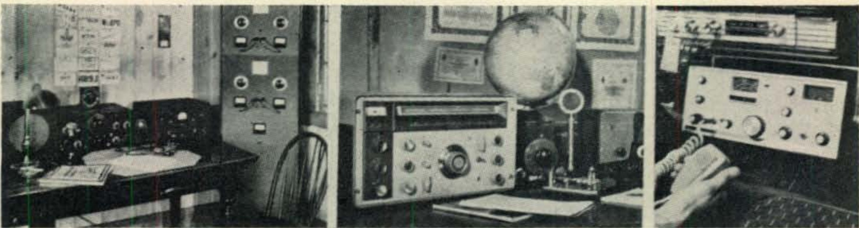
Left, a deluxe amateur station of the late 1930's; a NC-101X receiver, CRM oscilloscope, NTE exciter and the "600" transmitter. Center, National's "Dream Receiver", the NC-300, was probably the fastest selling amateur receiver during the mid 50's. The last photo is National's NCX-3, brought out in 1962. The NCX-3 with its accessory a.c. or d.c. power supplies is a complete 200 watt 80, 40, or 20 meter station.
